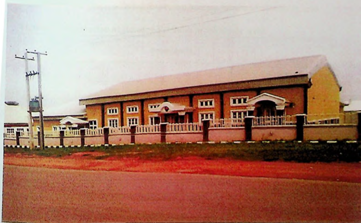
Plate 4.3: A Typical Good Housing Condition
