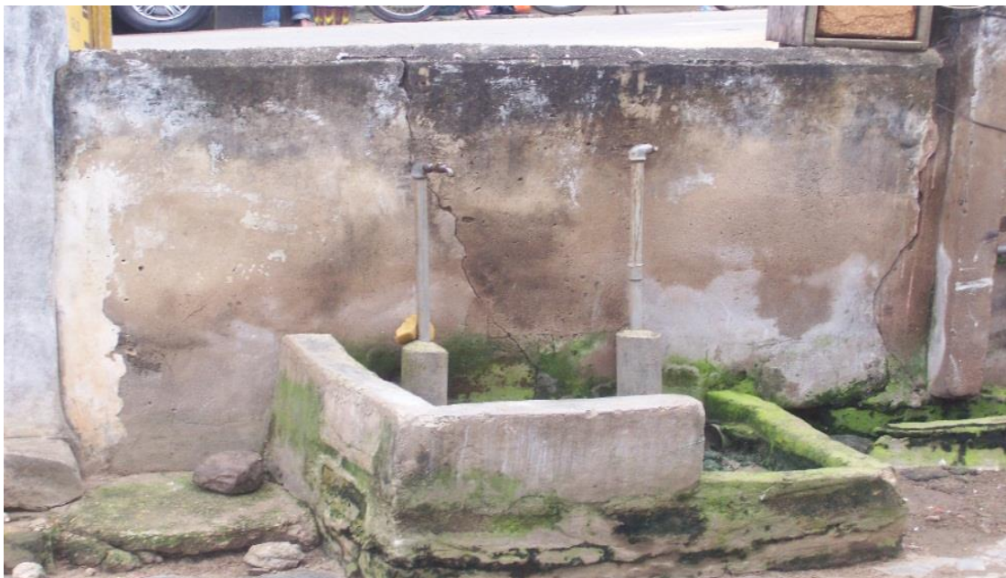
Plate 4.3: One of the Public Tap that is not functioning in Kubwa
