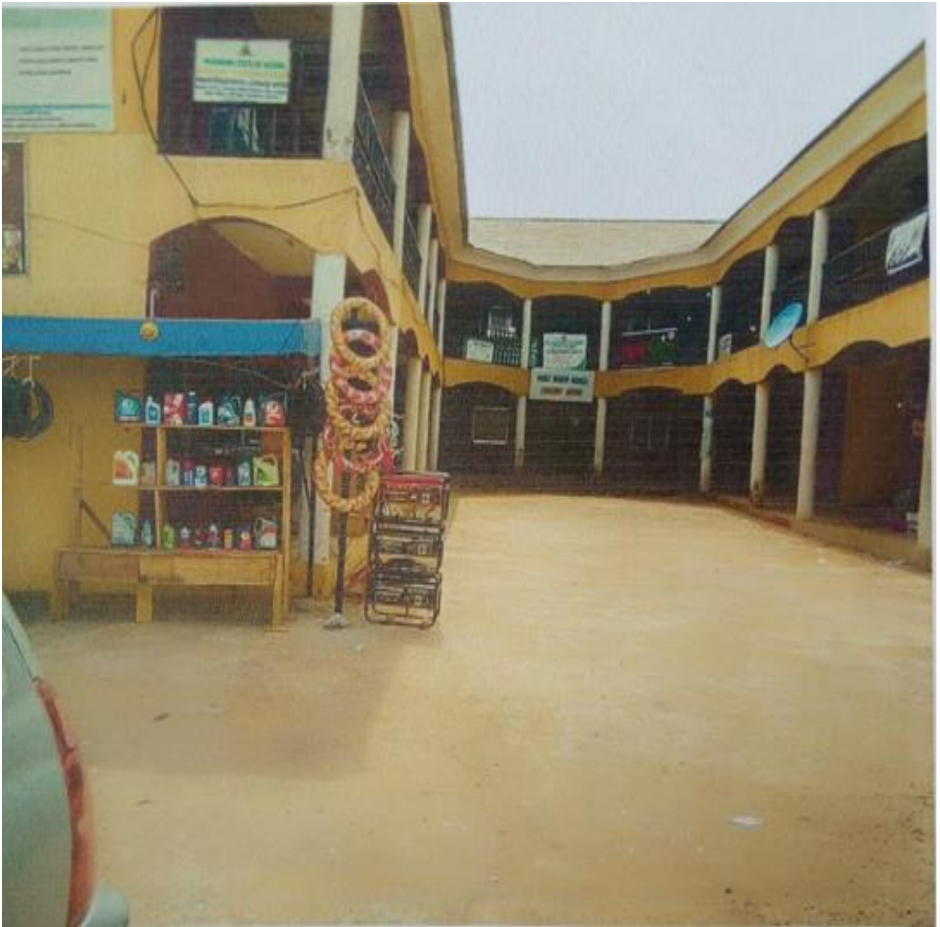
Plate 4.1. Picture showing commercial area at mararaba with generators working Source: Fieldwork, 2017
